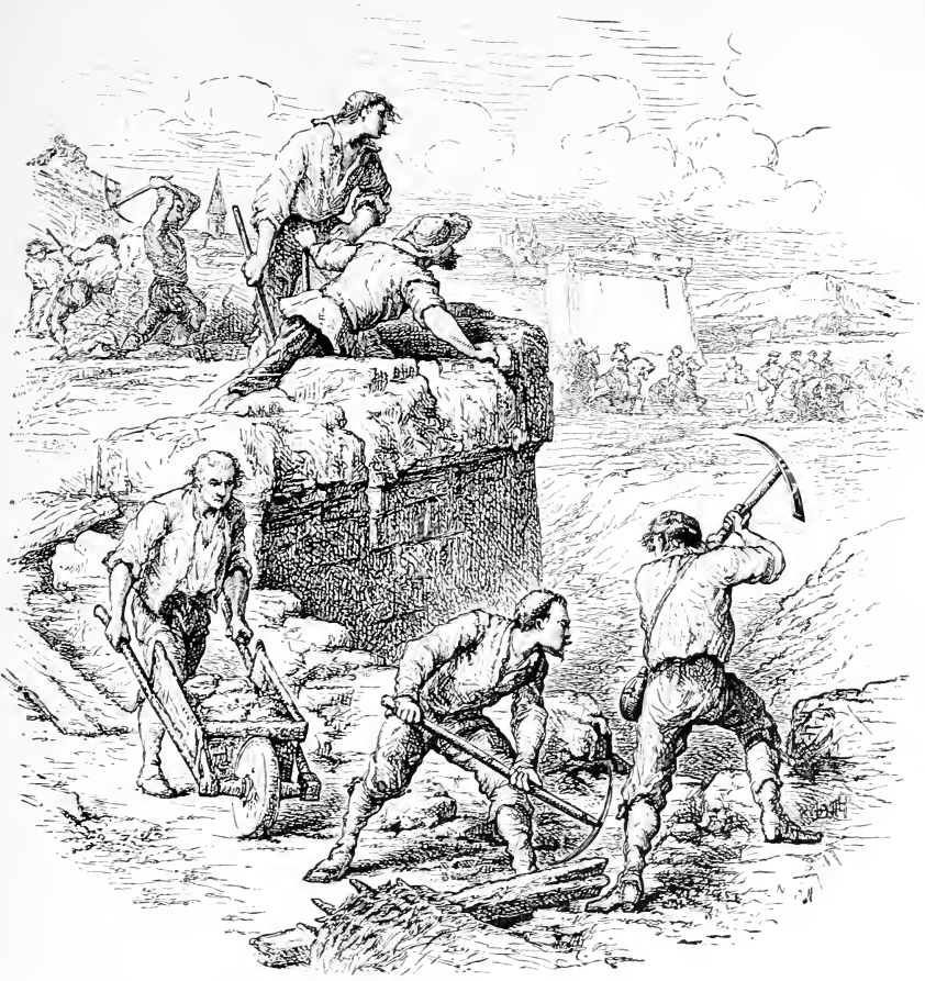
DEMOLISHING THE FORTIFICATIONS — Page 244.
